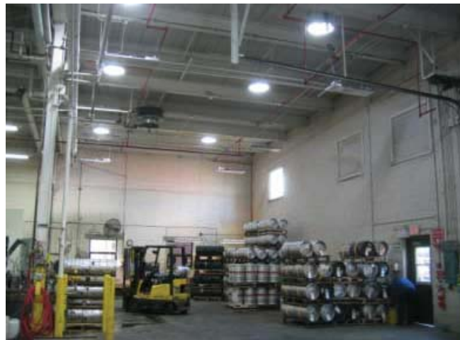
Solar Light Pipe 0 Watts
