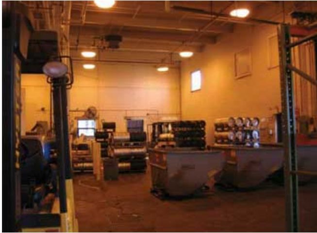
High Pressure Sodium 465 Watts
