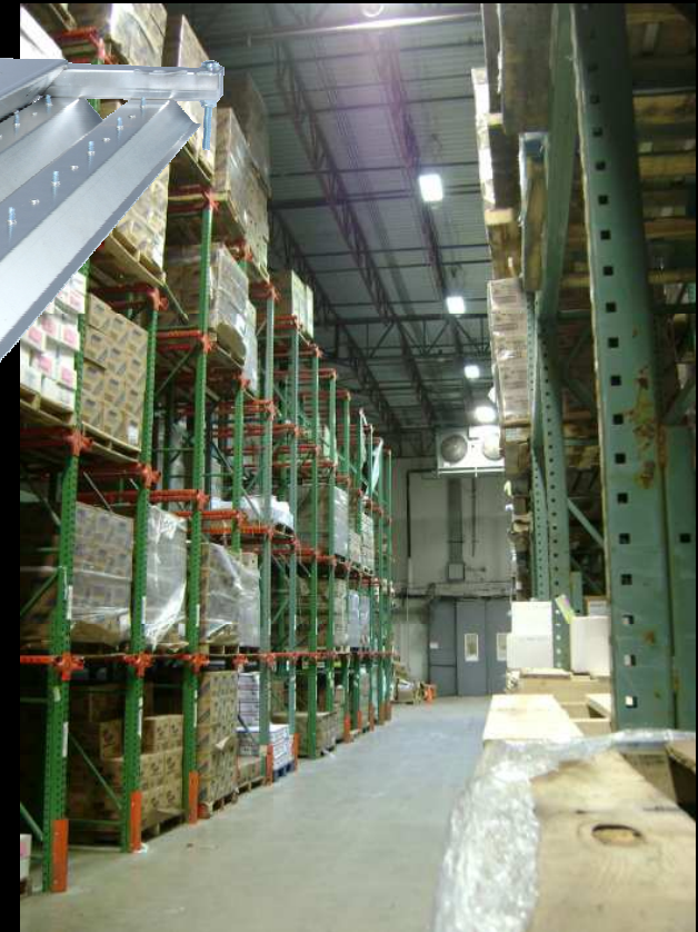
Orion LED 153 Watts 28 Footcandles
