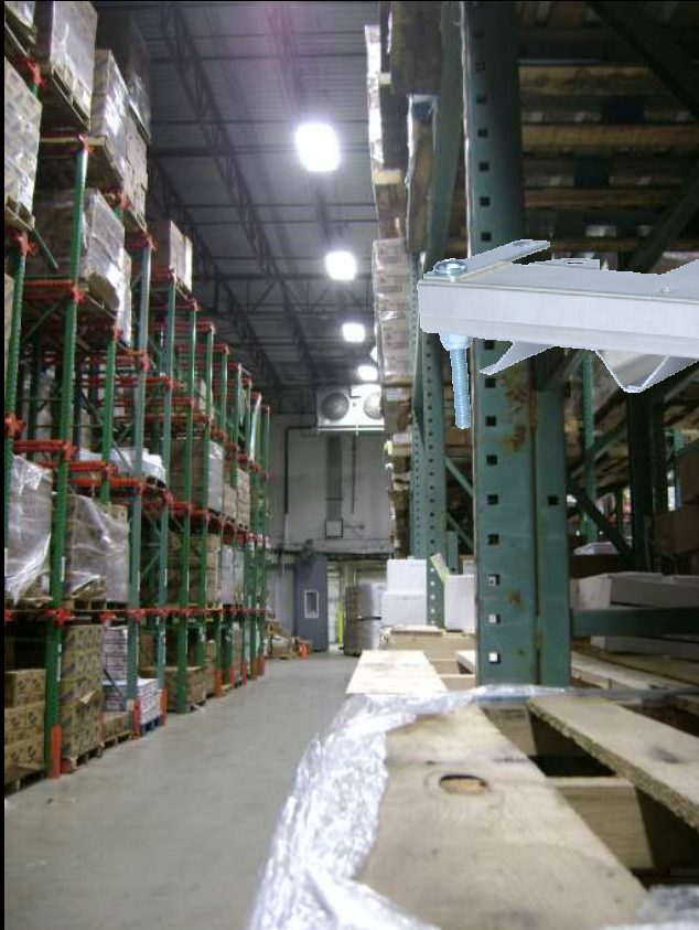
Orion Fluorescent 227 Watts 25 Footcandles
